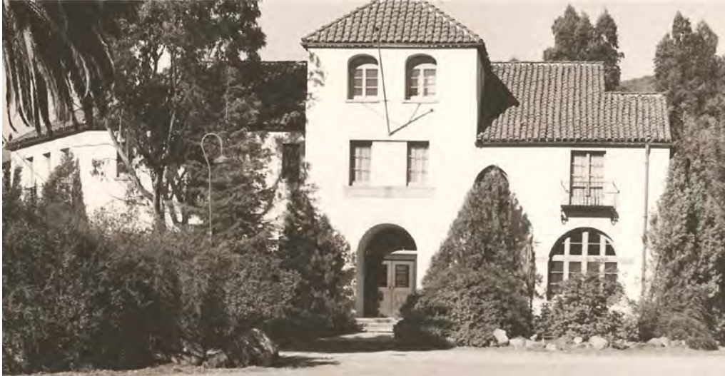
FIGURE 20 UNIT 1 FORMER CHAUFFEURS'/MAIDS' QUARTERS – c. 1946
