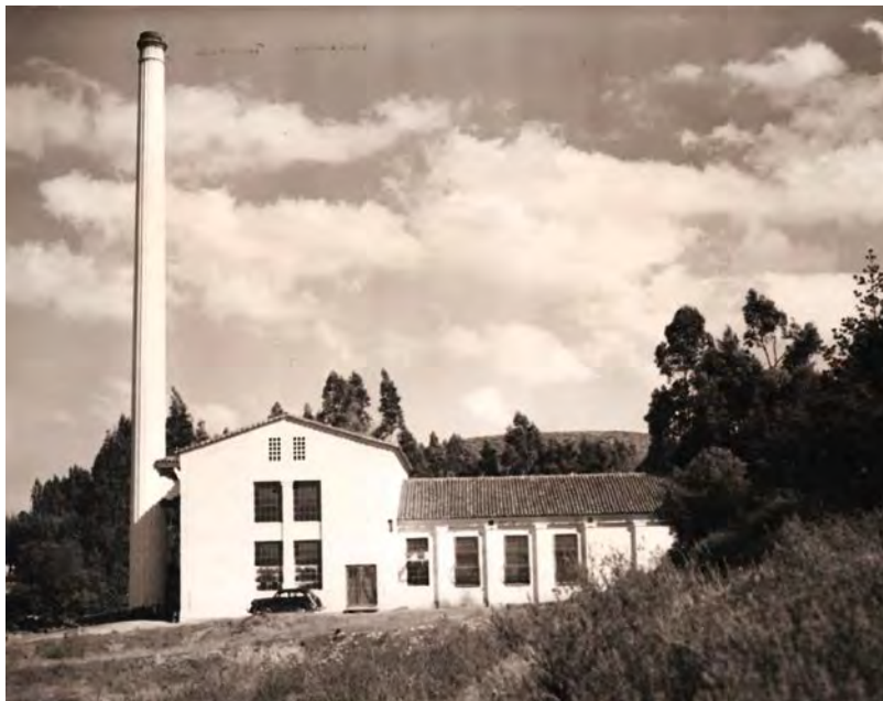
FIGURE 19 UNIT 1 POWER HOUSE – c. 1952
