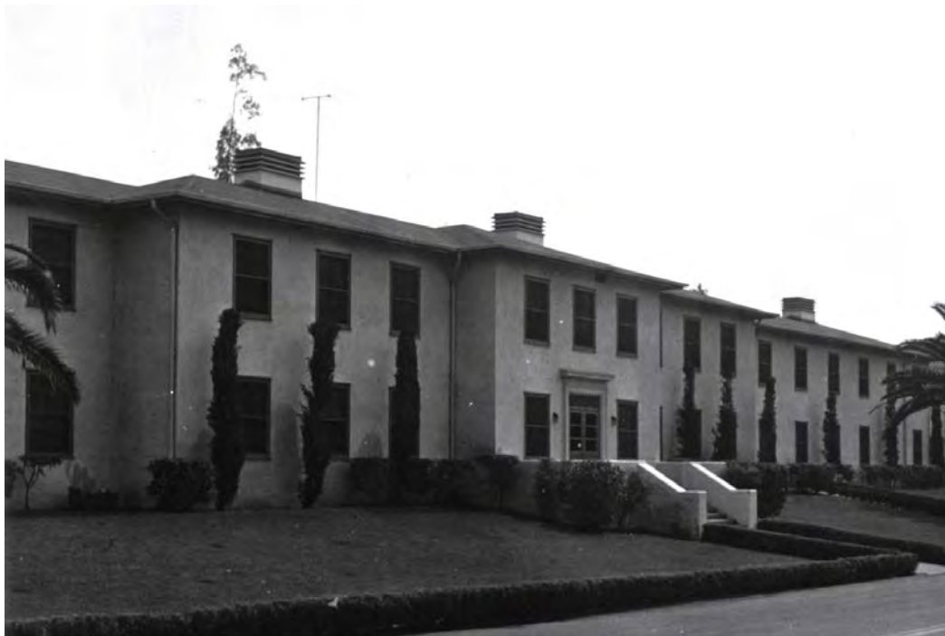
FIGURE 17 UNIT 1 WAVES' QUARTERS – c. 1946
