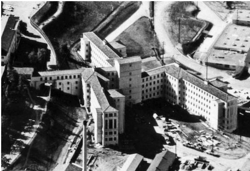
FIGURE 13 UNIT 1 ANNEX – c. 1943
