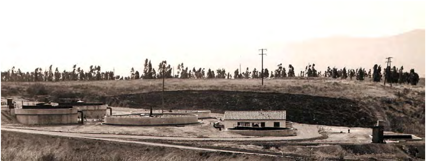
FIGURE 34 NAVAL HOSPITAL CORONA'S SEWAGE TREATMENT PLANT – c. 1946
