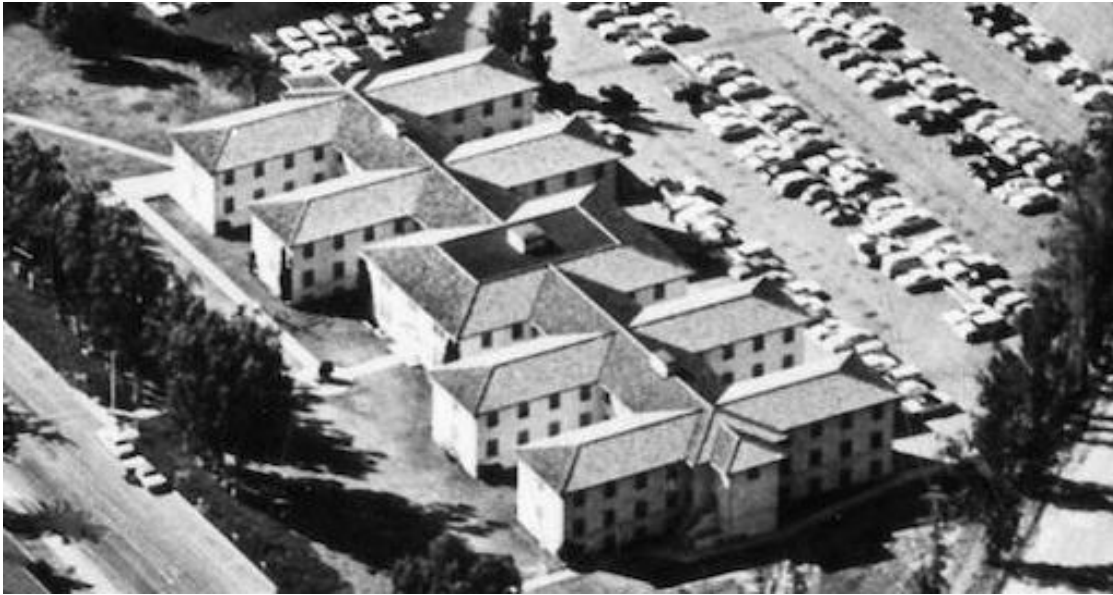
FIGURE 16 UNIT 1 CORPSMEN'S QUARTERS – c. 1946
