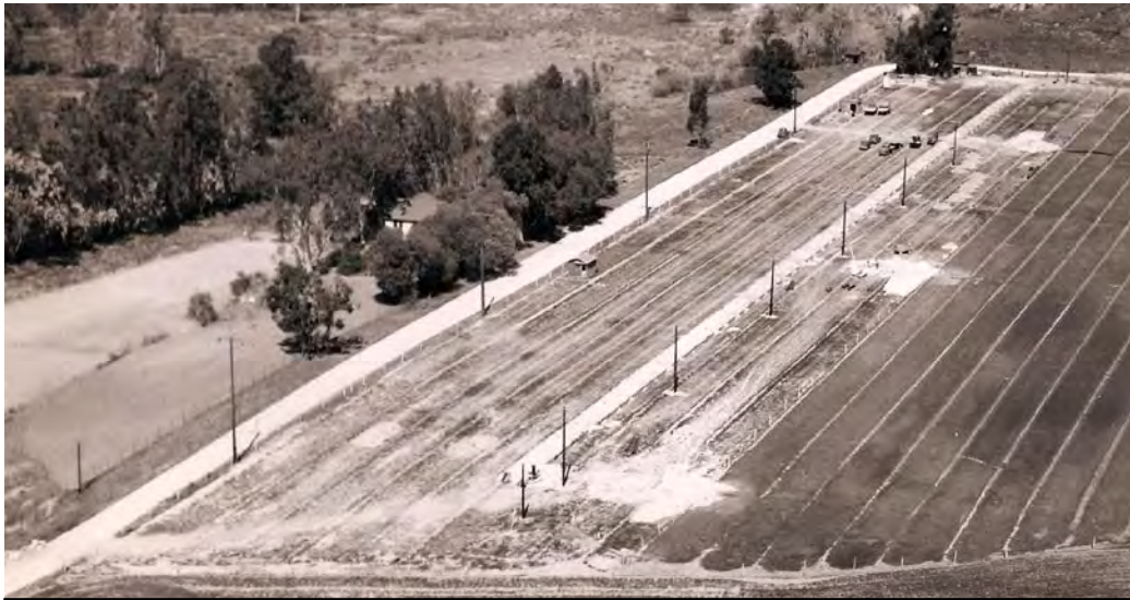
FIGURE 36 NAVAL HOSPITAL CORONA'S WATER WELLS – c. 1946
