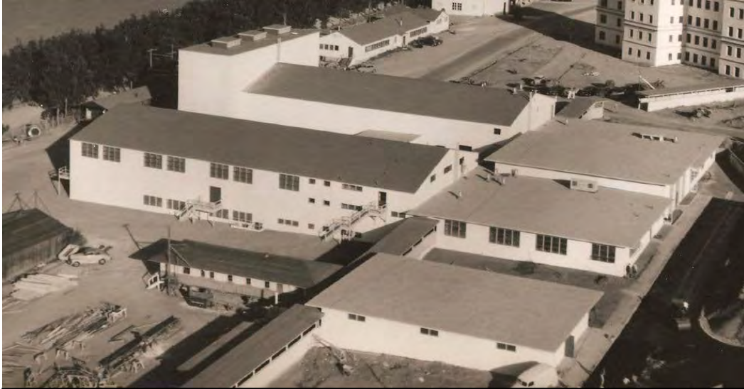
FIGURE 14 UNIT 1 GYM/THEATER COMPLEX – c. 1946
