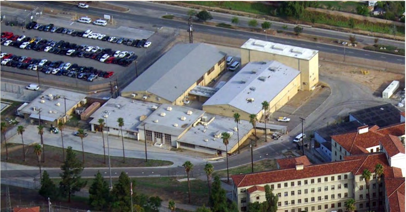
FIGURES 79-A and 79B ABOVE: GYM/THEATER COMPLEX 1946 BELOW: GYM/THEATER COMPLEX 2016 SOURCE: KEVIN BASH COLLECTION
