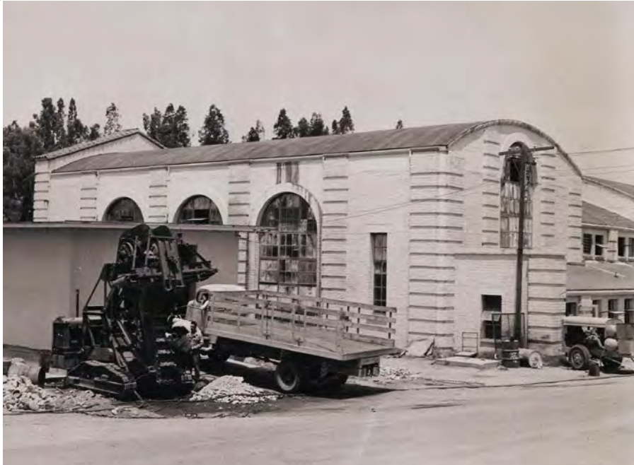
FIGURE 44 LAUNDRY PORTION OF GARAGE/LAUNDRY BUILDING (# 1, Fig. 43)
